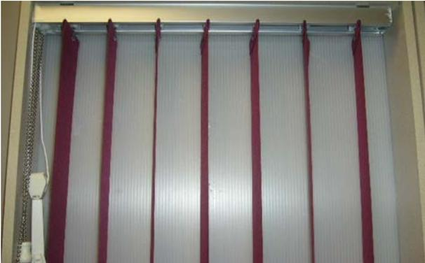
10. If spray lubricant is used on the pinion rod, remove louvers to prevent damage.
