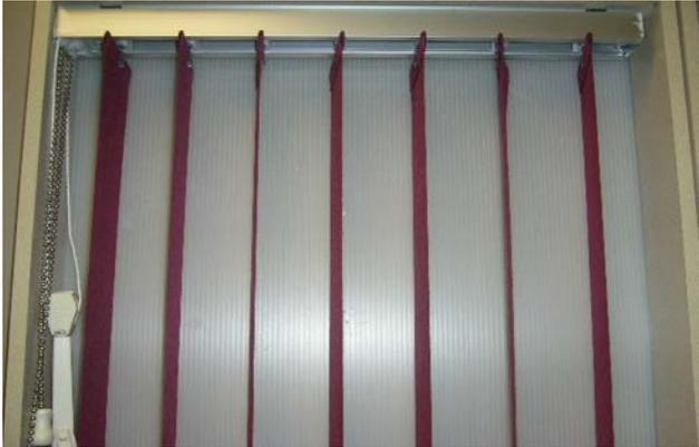
2. The headrail must be level both left to right and front to back. Use a level to ensure brackets are level. If not level, re-install the brackets.
