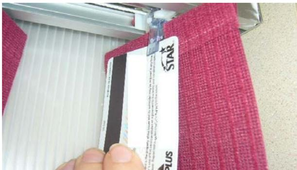
4. Remove the louver by pulling down on both the louver and the plastic card at the same time. Lay the louver on a clean flat surface. Repeat for all louvers.
