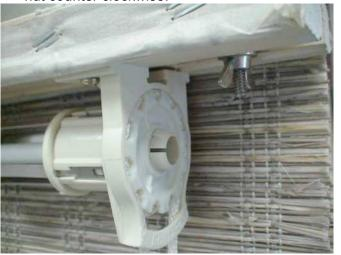
2. Remove screws from base of clutch.
